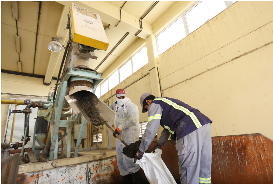
Treatment plant operators assorting the sludge into sacks
